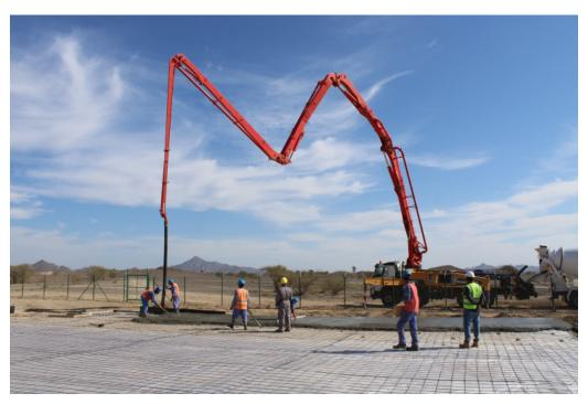
Picture 3: Dining area ground slab casting
