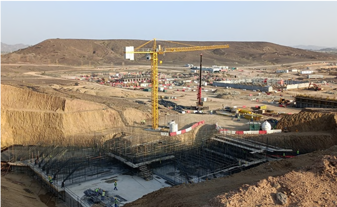
Copper-gold processing plant construction progress (late October 2022)
