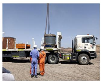
Pulp lifting (SAG mill)
