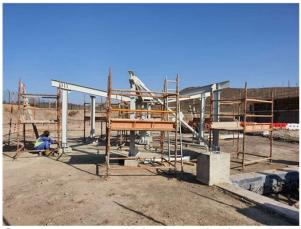
Copper concentrate thickener erection in progress
