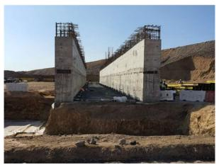
Crushed ore stockpile side walls completed
