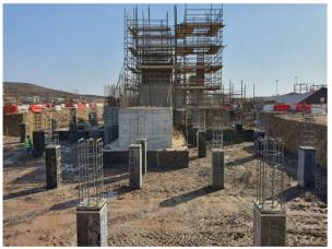
Mill area platform column foundation works
