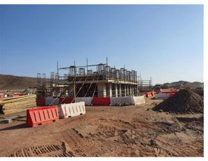
Rougher flotation cell foundation works
