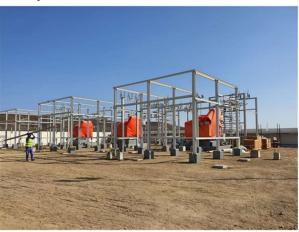
Primary substation - electrical works in progress
