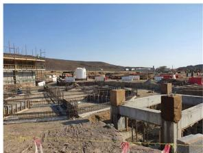
Tailing thickener backfilling works in progress
