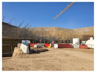
Primary crusher retaining wall under construction
