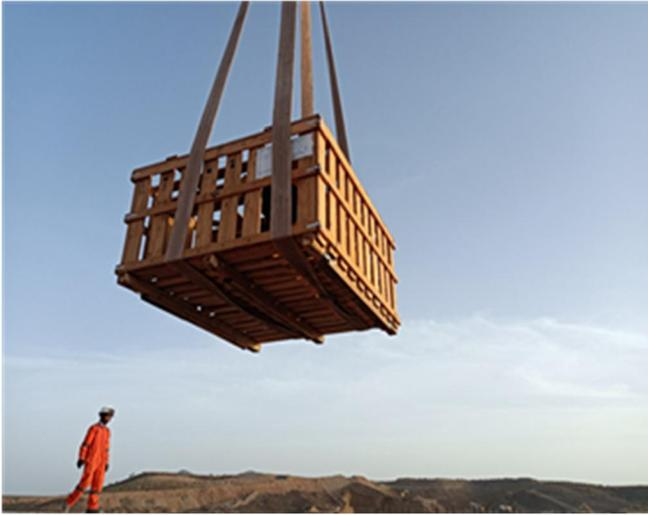
**Unloading LSS coupling guard (SAG mill)**
