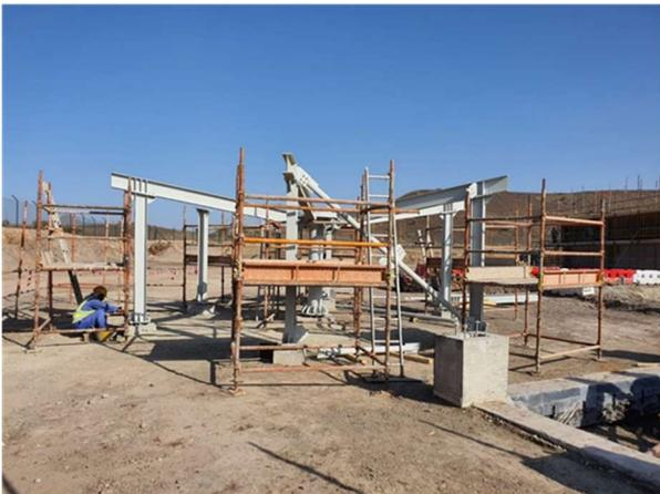
***Copper concentrate thickener erection in progress***
