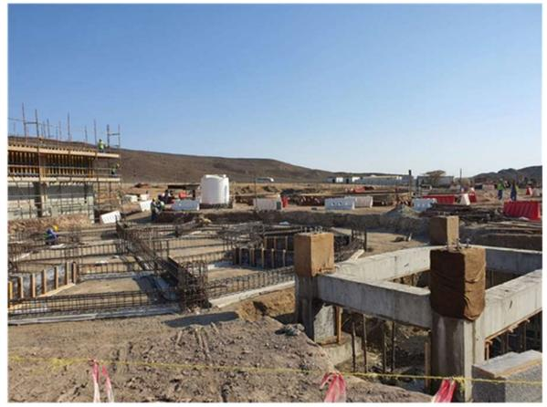
***Tailing thickener backfilling works in progress***
