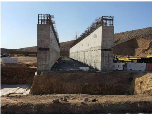
***Crushed ore stockpile side walls completed***
