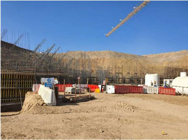
**Primary crusher retaining wall under construction**
