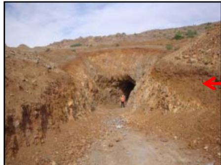
A half spiral decline dug in 2008 is wide enough to take regular trucks and loaders to sulphide mineralisation below the oxide cap, which covers most of the hill
