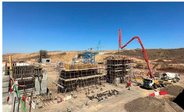
**Grinding mill foundation**
