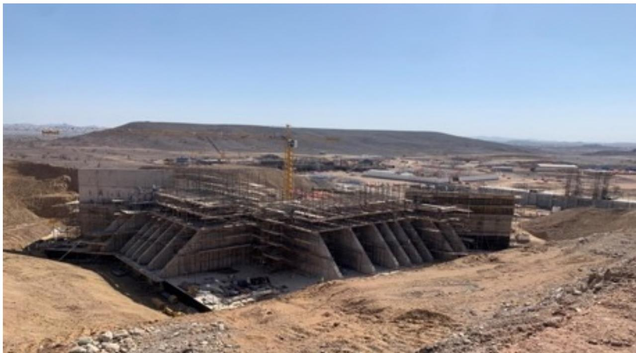
**Figure 1: Retention wall and primary crusher**
