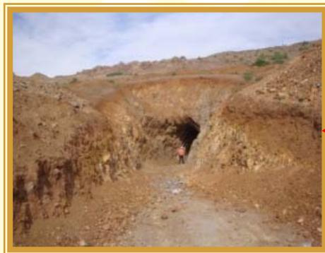
A half spiral decline dug in 2008 is wide enough to take regular trucks and loaders to sulphide mineralisation below the oxide cap which covers most of the hill
