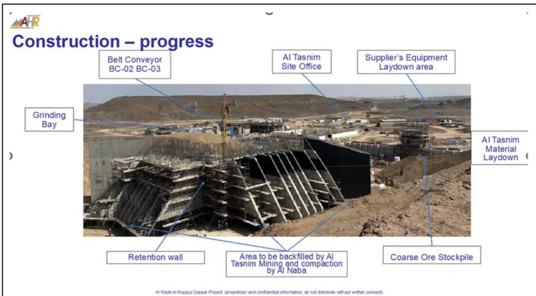
**Figure 4 Construction progress**
